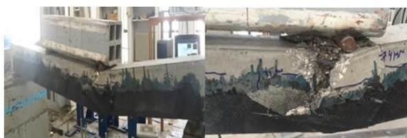
Fig. 11: The Load Displacement Curve of Beam F-60 and Its Crack Pattern.
