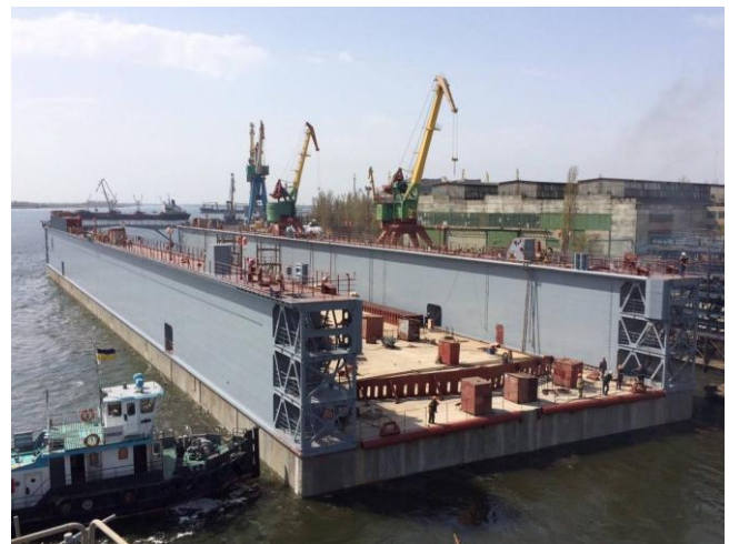
Fig. 1: Floating dock on a reinforced concrete pontoon, built at the Pallada plant
