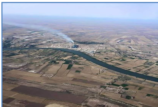
Fig. 1: Al-Zubaydiah Thermal Power Plant.
