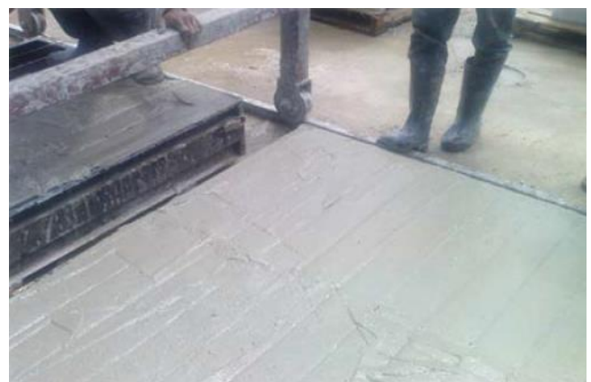
Fig. 2: Cellular mortar being poured to make blocks in steel molds
