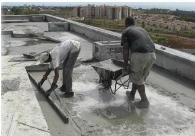
Fig. 1: Cellular mortar insulation screed for a multi-storey building in Mauritius
