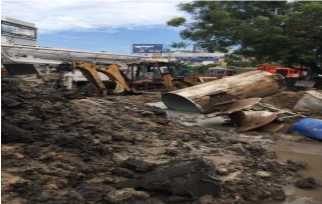
Fig. 3: Construction activities at Benz circle
