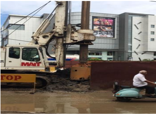
Fig. 4: Construction activities at Benz circle
