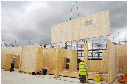
Fig. 2: Example of panel construction system [34].
