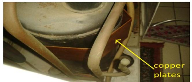
Fig. 4: Copper Plate for TEG Array mounted on the AC Compressor
