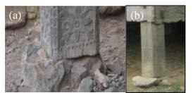
Fig. 2:(a). The umpak foundation system; (b) Foundation view
