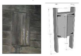
Fig. 5: Window view that does not have a grid for ventilation
