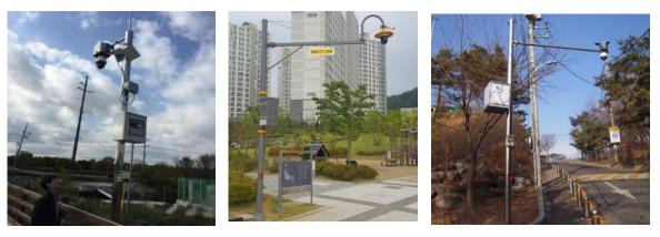
Figure 2. Control units installed to poles with CCTV cameras
