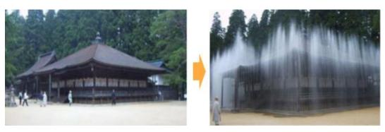
Figure2:.Fire Prevention water screen utility in Japan
