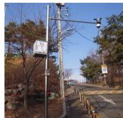
Figure 2:. Control units installed to poles with CCTV cameras
