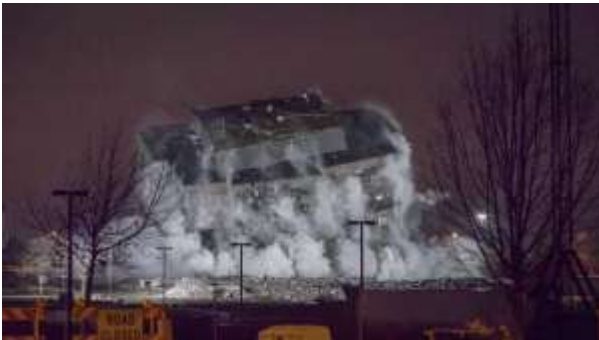
Figure 2: Demolition of building using explosive [4]
