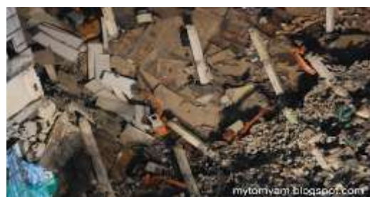
Figure 1 : An aerial view of the collapsed Jaya supermarket building[3]
