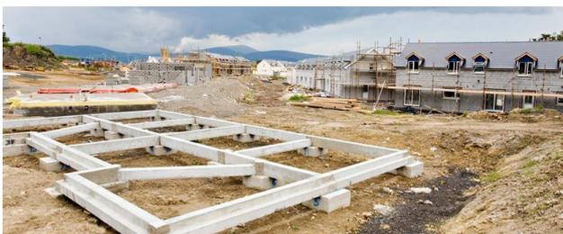
Figure 3. Precast foundation in Indonesia [13]
