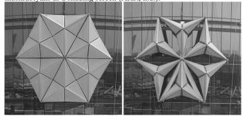
Fig. 1: Dynamic, sunlight-responding shading screen for Al Bahar Towers façade, reproduced from aedas.com/en.
