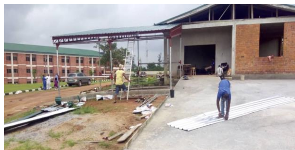
Plate 3: Roofing in Progress.
