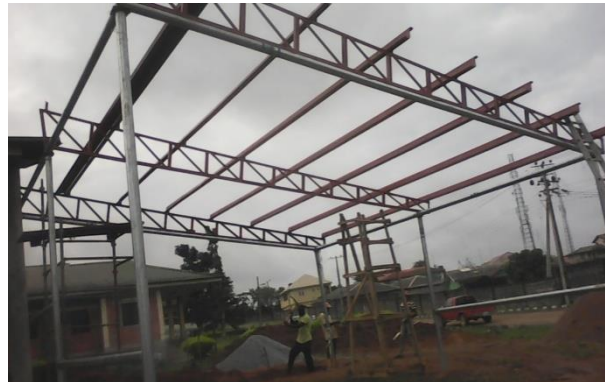
Plate 2: Installation of Trusses and Z Purlins.
