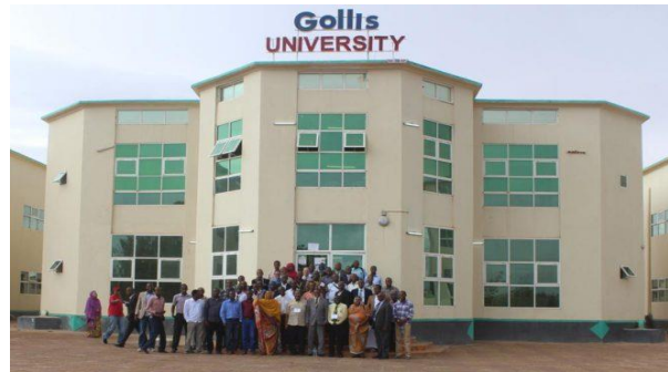
Fig. 7: Photography of Gollis University's Administrative Block.
