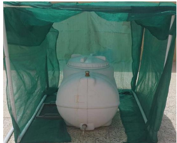
Fig. 2: Overhead Water Storage Tank with Shade (Case 3).
