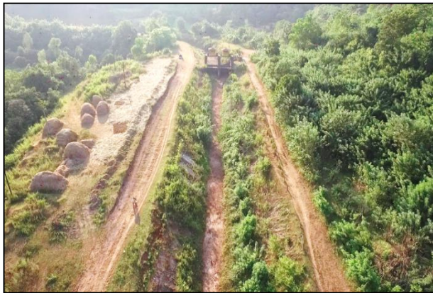
Photograph 1: Low Altitude Drone Image for Interpretation of Weeds, Siltation and Cracks.
