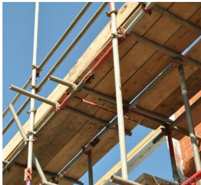
Fig. 1: General shape of scaffolding assembly at construction site
