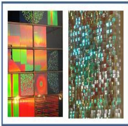
**Fig. 1:** a) Façade with holographic glazing Augenfeuer in Bonn. b) Sensitiles system light reflective polymer panels[14]
