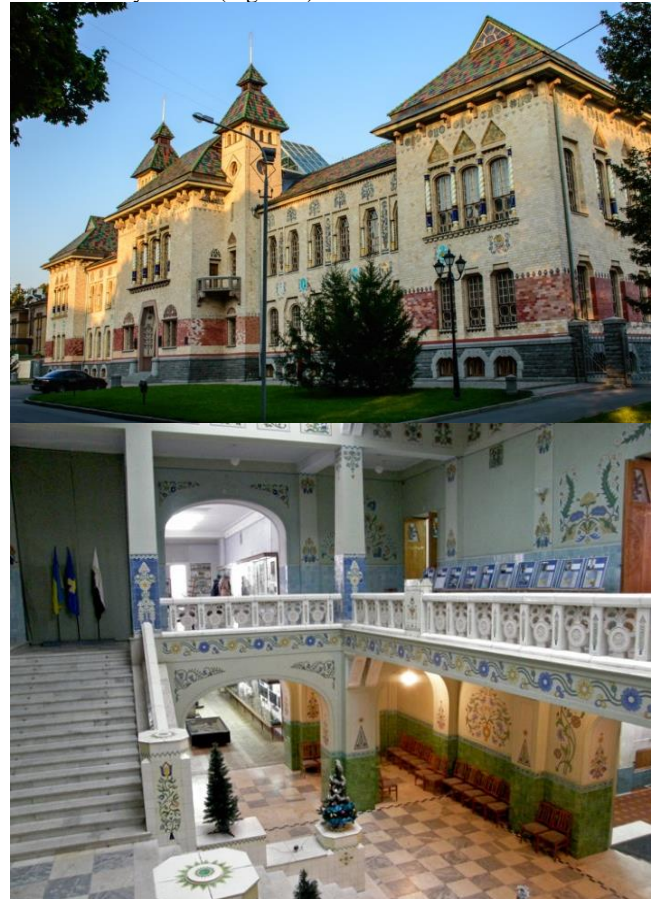
Fig. 2: Poltava Province Zemstvo, Ukraine, 1910 (Arch. V. Krychevsky). Main facade and central atrium.
