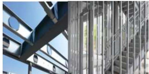
Fig. 1: Perforated Cold-Formed Steel Sections Used as Framing Members.
