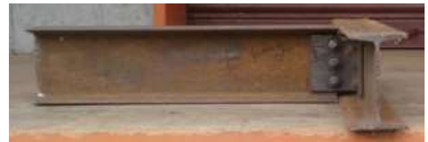
Fig. 5: Bolted Beam to Beam Connection.
