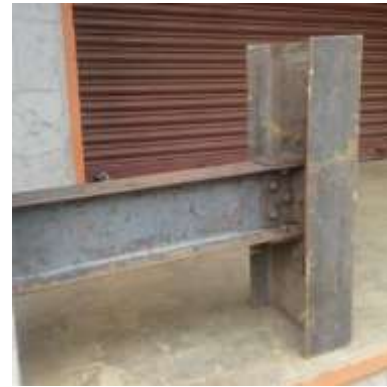
Fig. 3: Bolted Beam to Column Connection.
