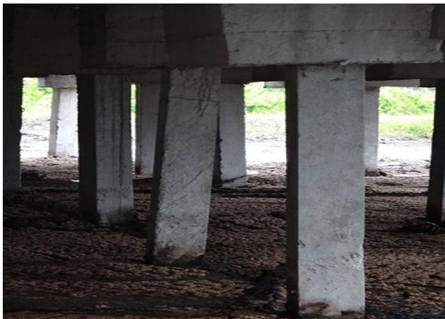
Fig. 5: Typical of existing inclination of pile
