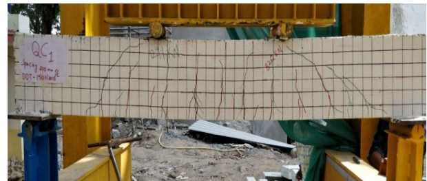
(a) Flexural and shear cracks in BWSC-1
