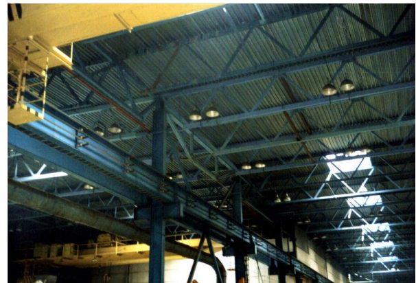
Fig.15. Trussing beam-truss L=12m. Experimental research factory, Lviv, Ukraine
