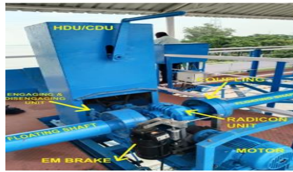
Fig. 2: Barrage Gate Lifting Mechanism.
