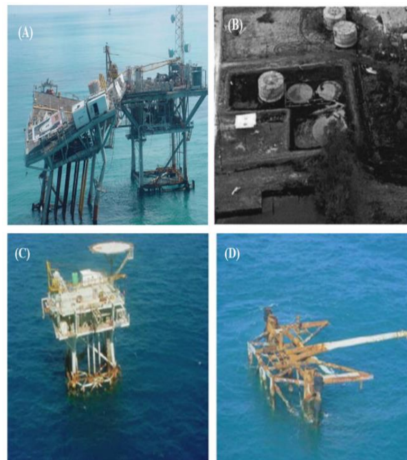
Fig. 2: Examples of Extreme Storm Impacts on Coastal and Offshore Petroleum Infrastructure.
