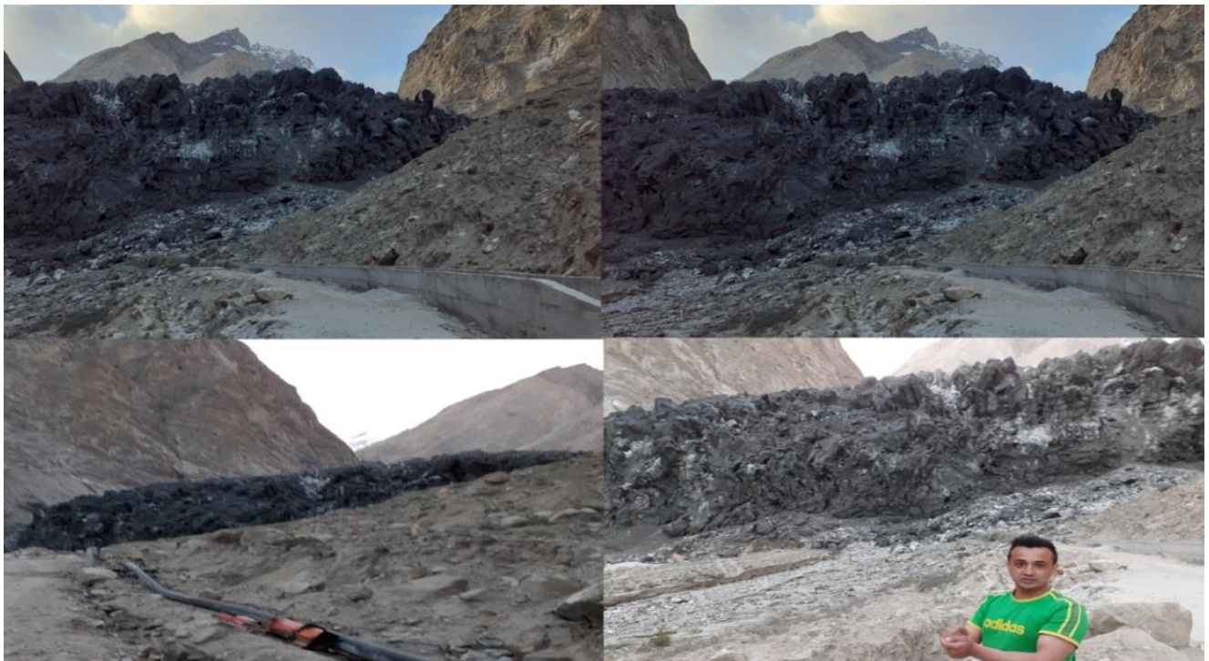
Fig. 4: Field Photos of Shispar Glacier Tongue. These Pictures Have Taken at May 10 2019, Show the Advanced Tongue of Shispar Glacier and Also Show the Power House and Irrigation Channels Damages.
